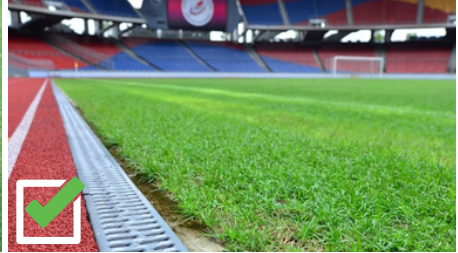
Proper drainage cover
