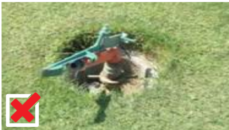
Exposed irrigation head
